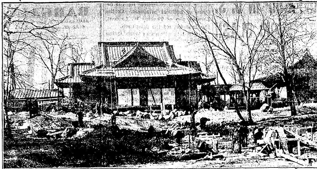
The picturesque Japanese buildings of the World's Fair of 1893, which have stood on Wooded island in Jackson park for forty-one years, are being restored by the south park board with the aid of public works administration funds.
